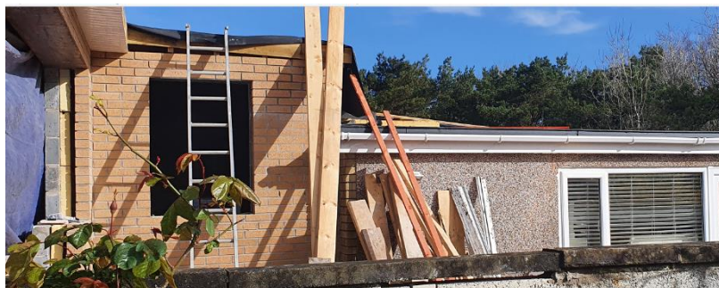
Fig. 5 – Relationship between the bedroom window and 40, Hunters Ridge
